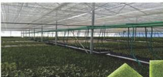
Nursery specializes in production of potted plants, ranging from Protea cultivars to Geraldton Wax Flowers for garden centres and landscapers. 94 movable tables of 1.6m X 5m are maintained at a constant 23°C soil temperature, utilizing bulk hot water storage heated by solar panels and heat pumps as supplement.
