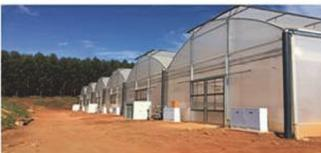
2 880 m<sup>2</sup> of floor area consisting of 6 bays, 480 m<sup>2</sup> each, kept at variable temperatures ranging from 15°C to 35°C. An accuracy of 1°C variance is maintained. Utilizing heat pump technology, the total hourly load of 438 kWatt was reduced to an input of 132 kWatt. Total potential saving for Mondi is estimated at 3 600 kWatt/ day
