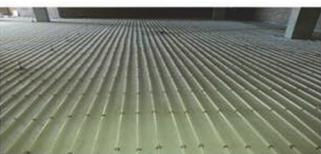
By a process of heat recovery, free energy is harvested from the refrigeration plant and circulated through PEX tubes to the cold room floors. Due to temperatures ranging far below 0°C, the free heat energy is utilized to prevent the floor from freezing up and ultimately cracking. Electrical elements are installed as back-up.
